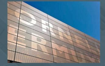
Contrast can be achieved on an expanded metal mesh by simply rotating the mesh upside down.
