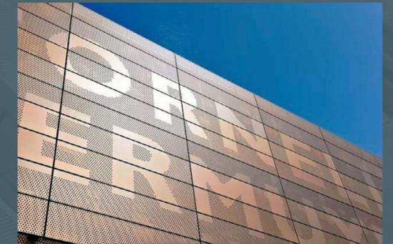
Contrast can be achieved on an expanded metal mesh by simply rotating the mesh upside down.
